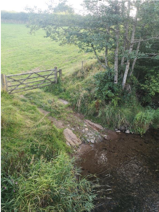
South Bank Revetments
