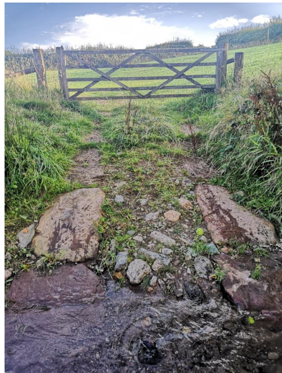
North Bank Revetments
